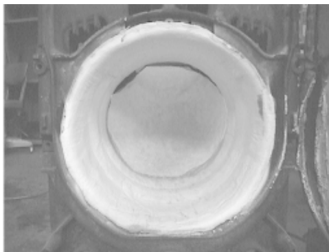
Size 140 or 235 with a new liner installed
